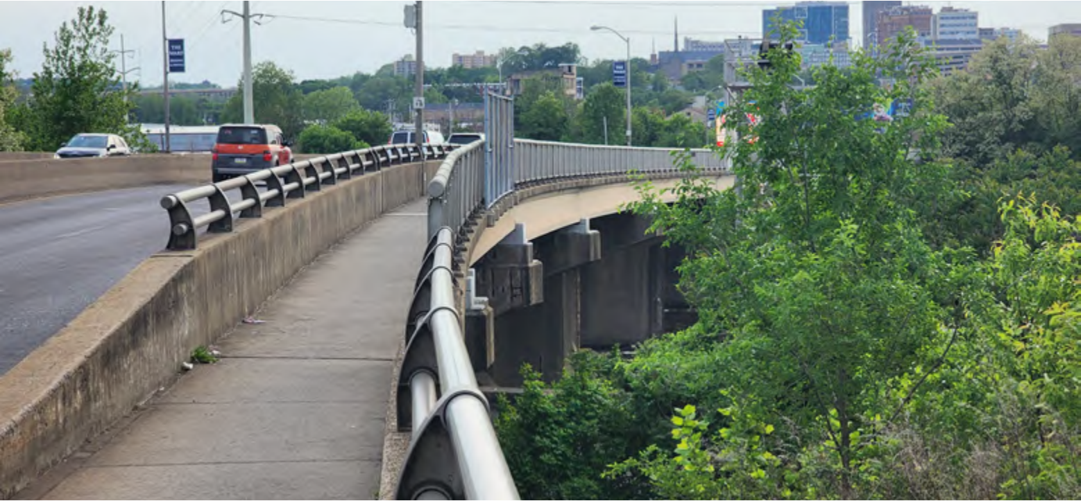
Hamilton Street Bridge over the Lehigh River
