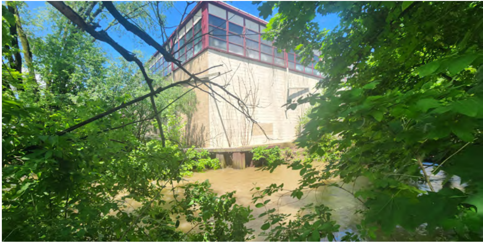
Derelict building constructed into Cedar Creek
